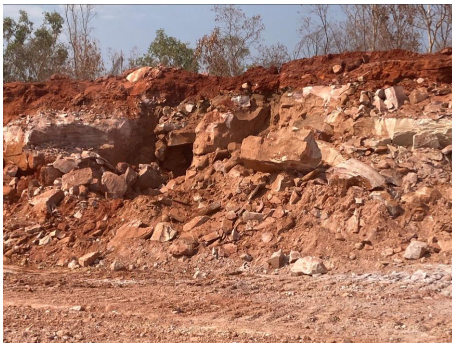
Figure 4: Excavation face noting Pindan Sands and Melligo Sandstone intersections
